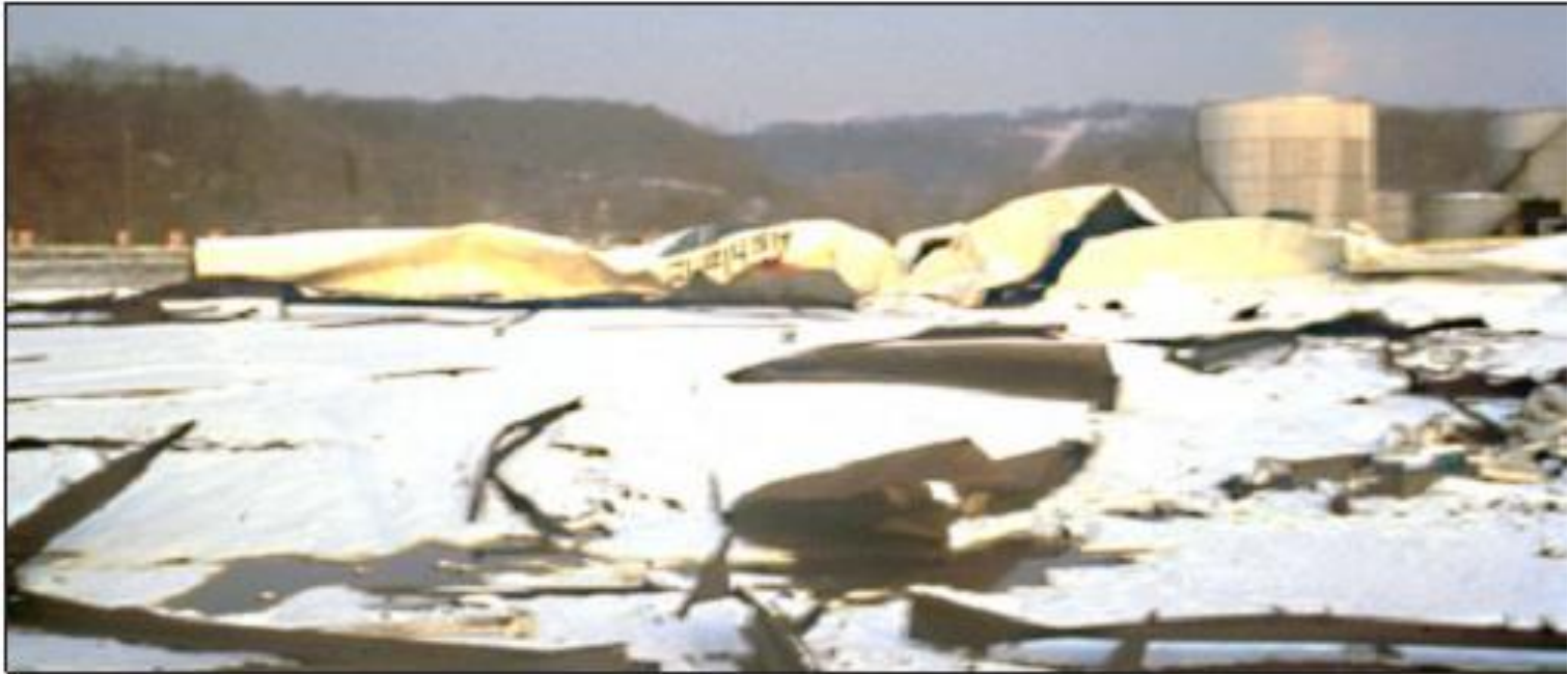
Figure 1. Collapsed storage tank.
